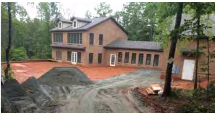
Michael Schlitz Home Status: Under Construction
